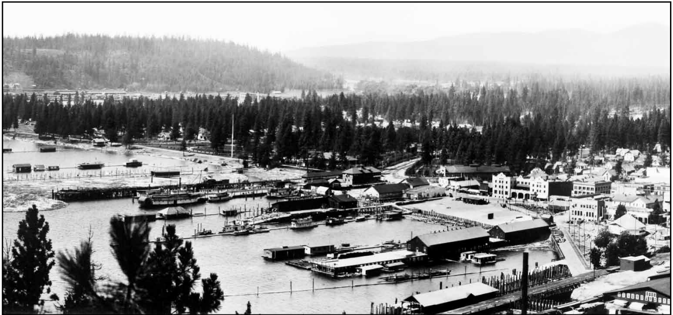
Coeur d'Alene waterfront after 1908 but before 1910. Notice the cribbing holding in the fill in front of the Hotel Idaho. At this time 1st St. does not extend to Sherman Ave. When the Milwaukee Railroad built its depot and tracks in front of the hotel even more fill was added into the lake.
